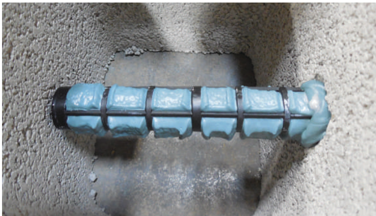
Hollow CMU Install with Opti-Mesh Screen
