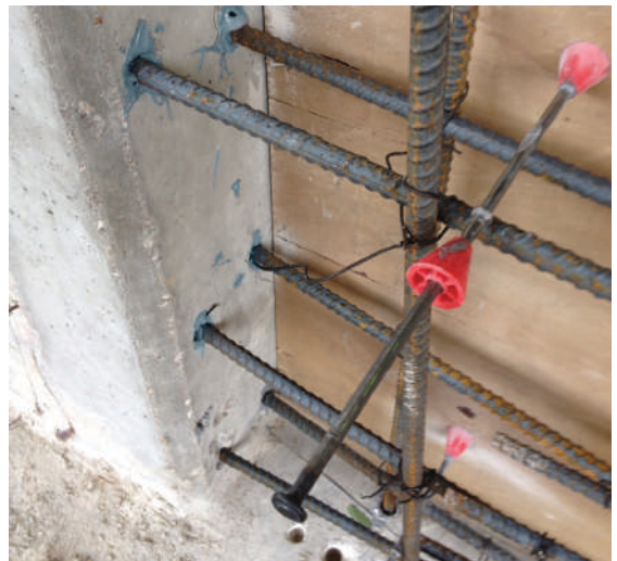
Rebar Wall Extension
